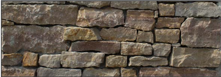
COLUMBIA PLATINUM HAMMER BROKE
